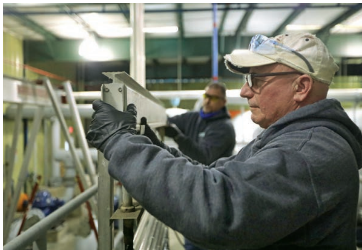
Boyle performs maintenance on the TrojanUV3000 disinfection system.
