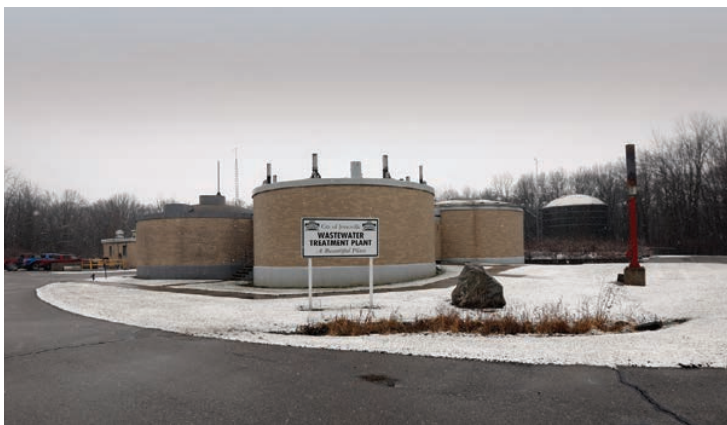
The Jonesville Wastewater Treatment Plant was upgraded in 2005 with 0.61 mgd design capacity; it now has a 0.34 mgd average flow.
